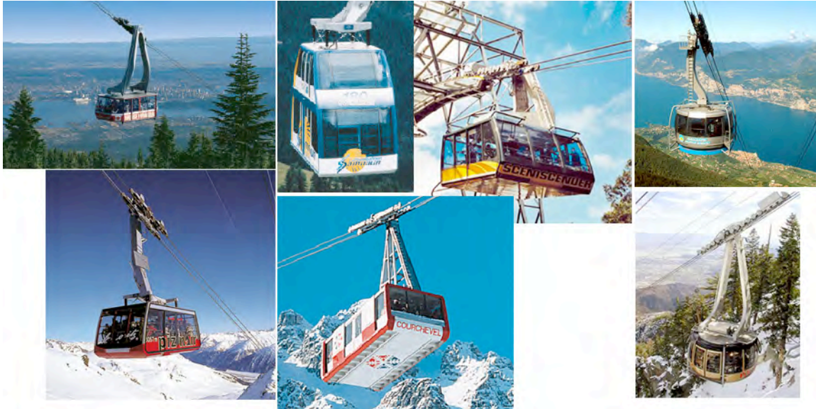
Aerial tramways provide cost effective, relatively low impact and efficient mountain transportation for skiers and tourists throughout the world. Clockwise from top left: (1) Grouse Mountain, Canada, (2) Samnaun-Alp Trida, Switzerland, (3) Katoomba, Australia, (4) Palm Springs, U.S.A., (5) Courchevel, France, (6) St. Moritz, Switzerland.
